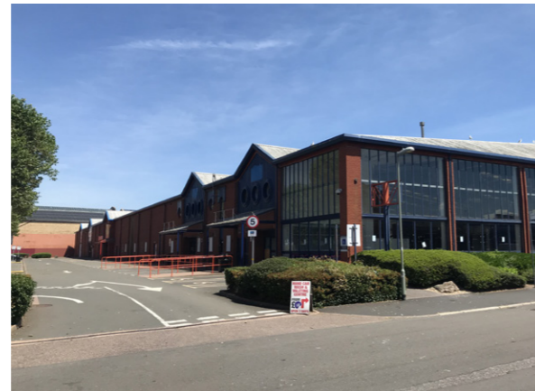
Vehicular Access onto Water Lane
