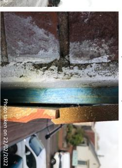
roof – note, breathable membrane lining Eaves roof space, inside south-western elevation monopitched
