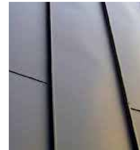
Standing seam aluminium cladding RAL7012
