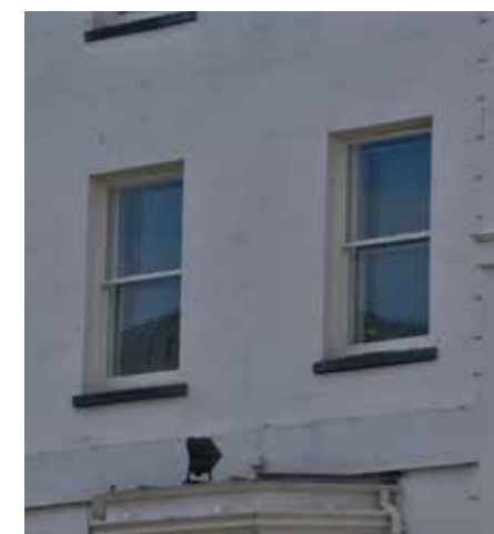
White timber sash window with no glazing bars; black cills
