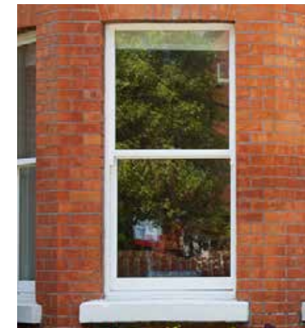
White timber sash window with no glazing bars
