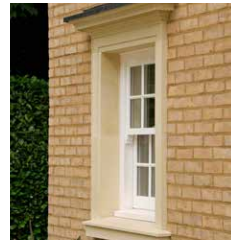
Foamstone window surround or similar; colour to match facade
