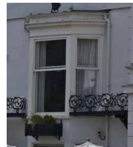
White bay timber sash window with no glazing bars
