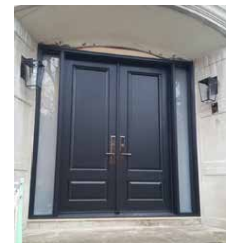
RAL7016 timber composite panel doors
