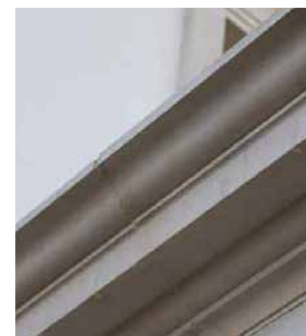
Foamstone cornice or similar; colour to match facade render
