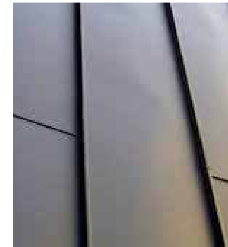
Standing seam aluminium cladding RAL7012
