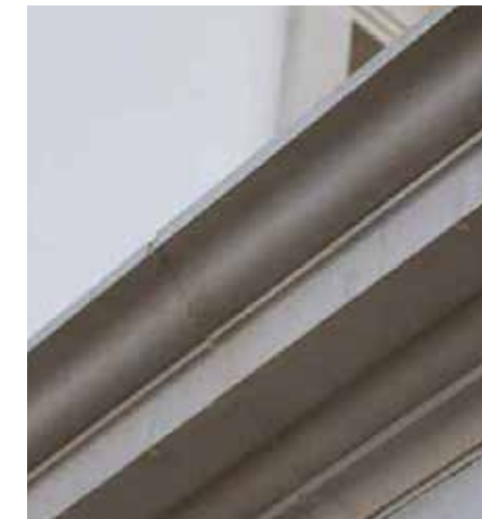
Foamstone cornice or similar; colour to match facade render
