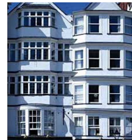
White timber frame windows, render and detailing restored
