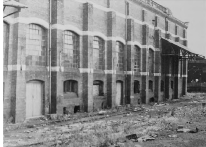
The rear of the boiler house was served by large windows
