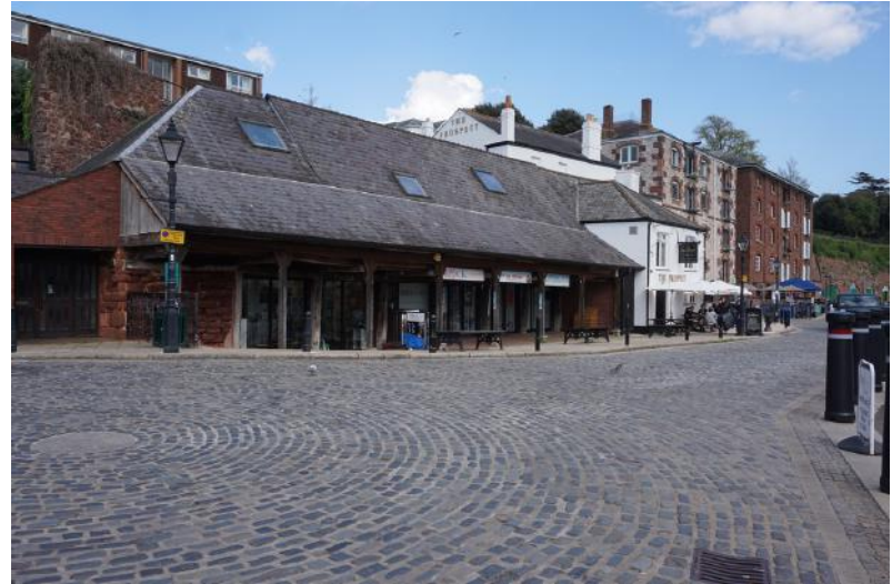
The Quay, Grade I listed, is an early and well-preserved transit shed.
