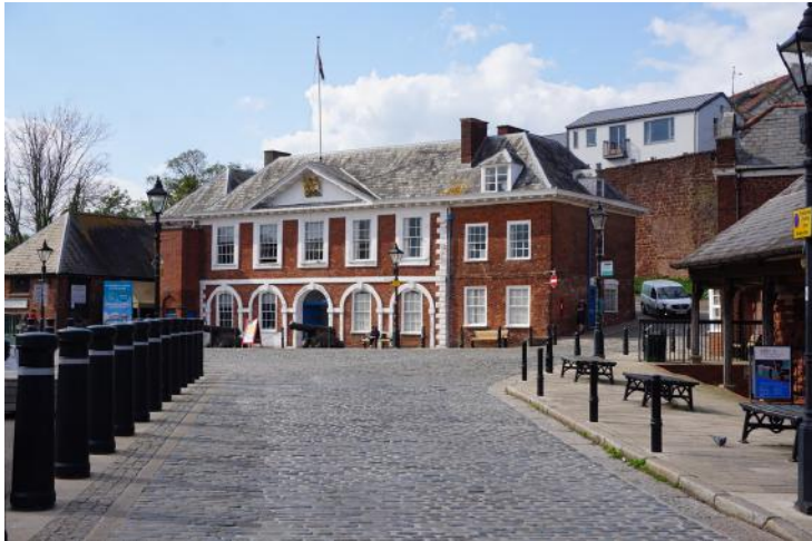
The grade I listed 17 th century Custom House is the centrepiece of the Quay area but the group value of the ensemble is also high.
