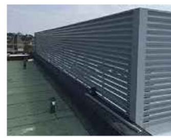
18 - Louvred Plant Screen Colour: RAL 7045
