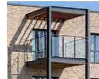
15 - Steel Balcony and Frame Colour: RAL 7012 & 7045
