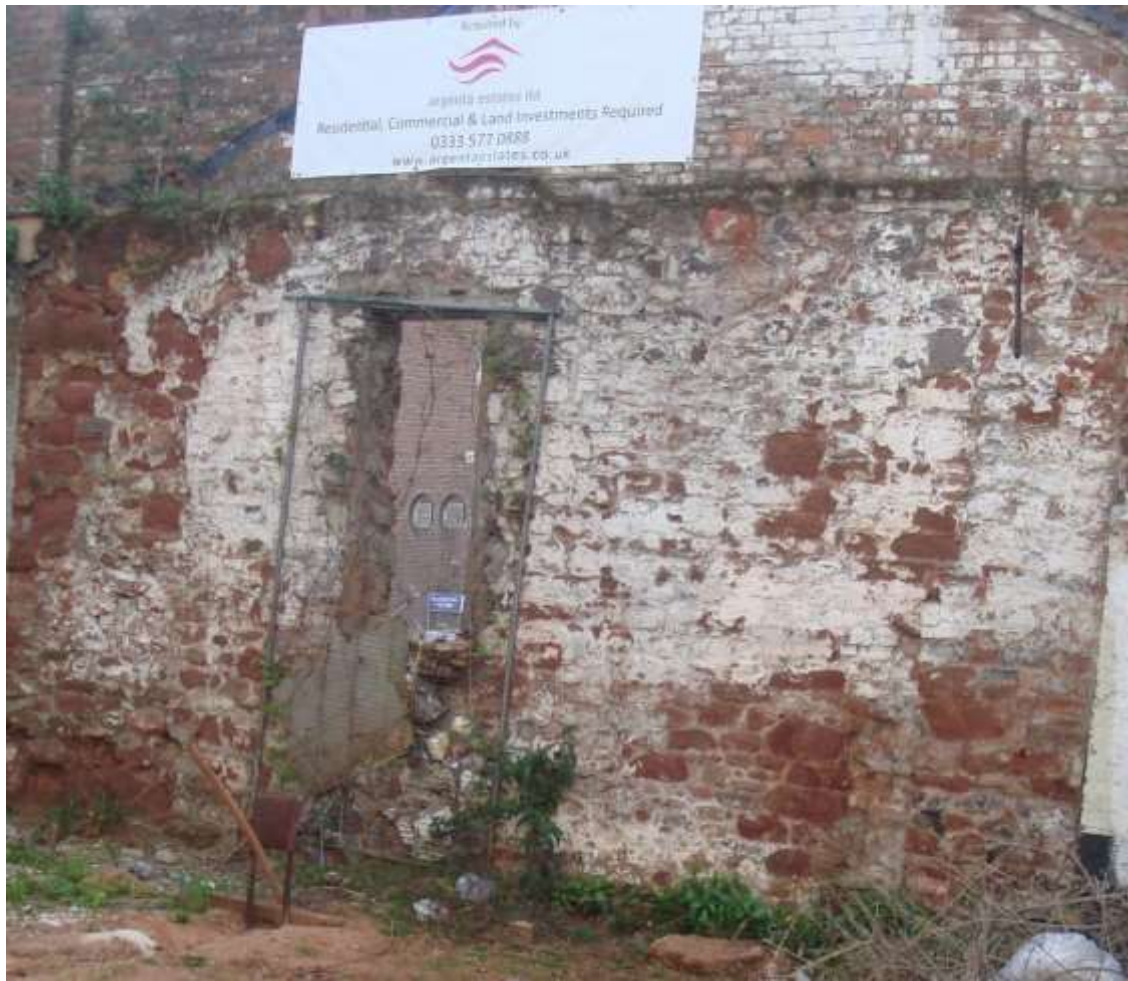
Photo 4: Detail of the rear (boundary) wall at 30-32 Longbrook Street showing the pitched roof 'scar' of the later garage against the brick heightening of the 19 th century.
