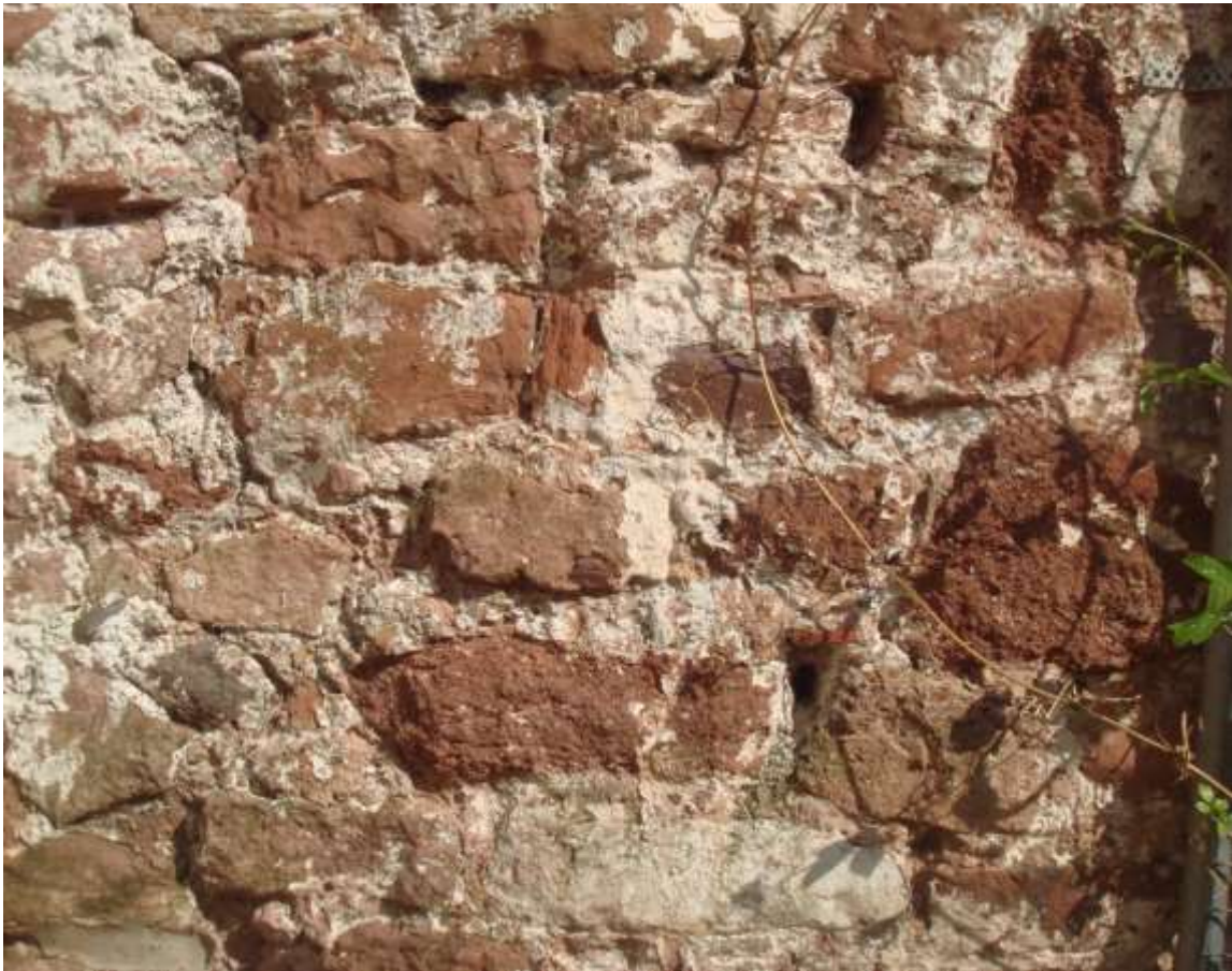
Photo 5: Detail of the rear (boundary) wall at 30-32 Longbrook Street showing the Heavitree and red sandstone blocks of the wall fabric.
