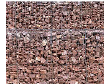
05 - Gabion Retaining Walls
