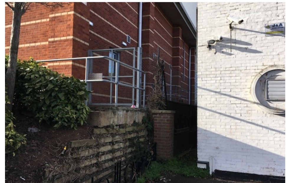
Photo showing the level difference between the two sites, with the existing red brick Aldi building to the left, and the site boundary to the garage building to the north
