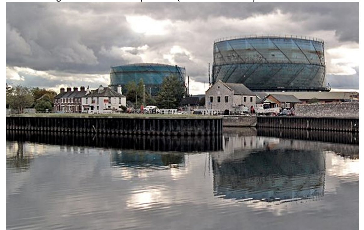
The Gasworks at Haven Banks - 2004
