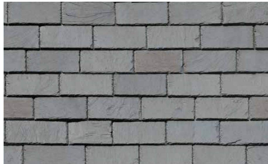
Natural Slate Roof.
