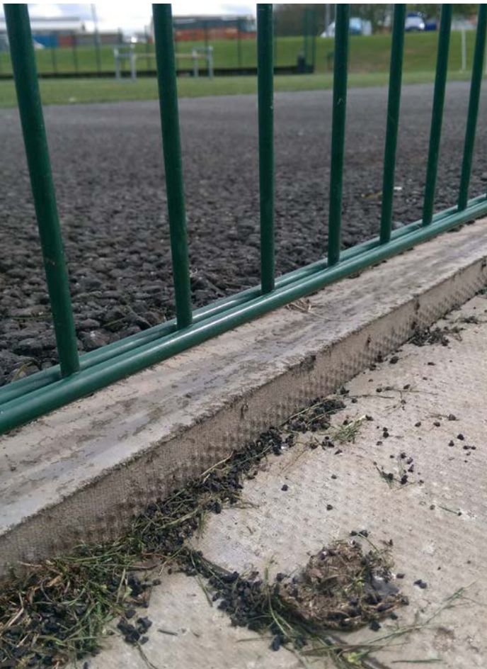
Figure 6. Rubber granules scattered on the outside edge of a pitch - the fence is open at the base allowing granules to escape easily
