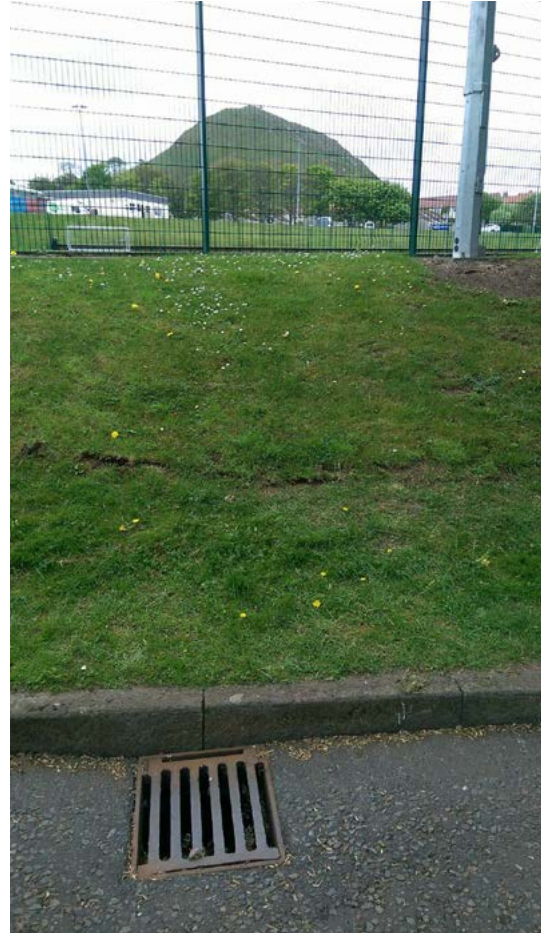
Figure 5. A pitch that is elevated to its surroundings, and close to an open gutter represents a risk of granules escaping directly to storm water
