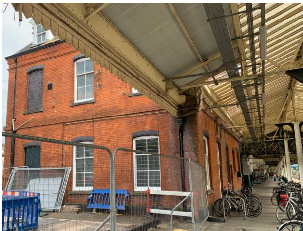
Figure 6 : Section of canopy to be adapted and made good once building has been demolished from the front
