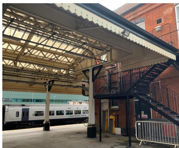
Figure 4 : Section of canopy to be removed to facilitate the platform extension supporting post in exclusion zone
