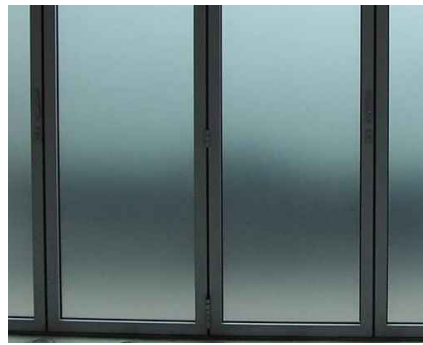
09 - Obscured Window Glazing
