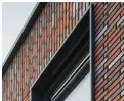
13 - PPC Aluminium External Window and Door Reveals Colour: RAL 7012
