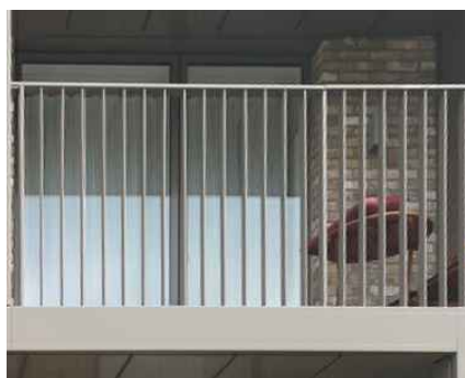
17 - Metal Balustrade Colour: RAL 7012
