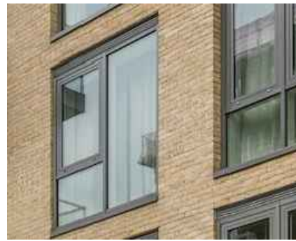
07 - PPC Aluminium External Window and Door Frames Colour: RAL 7012
