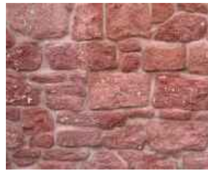
04 - Facing Stonework Colour: Red Sandstone
