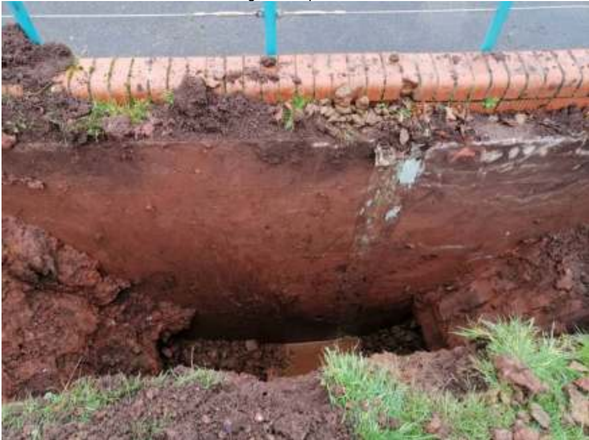
TP05 – retaining wall.
