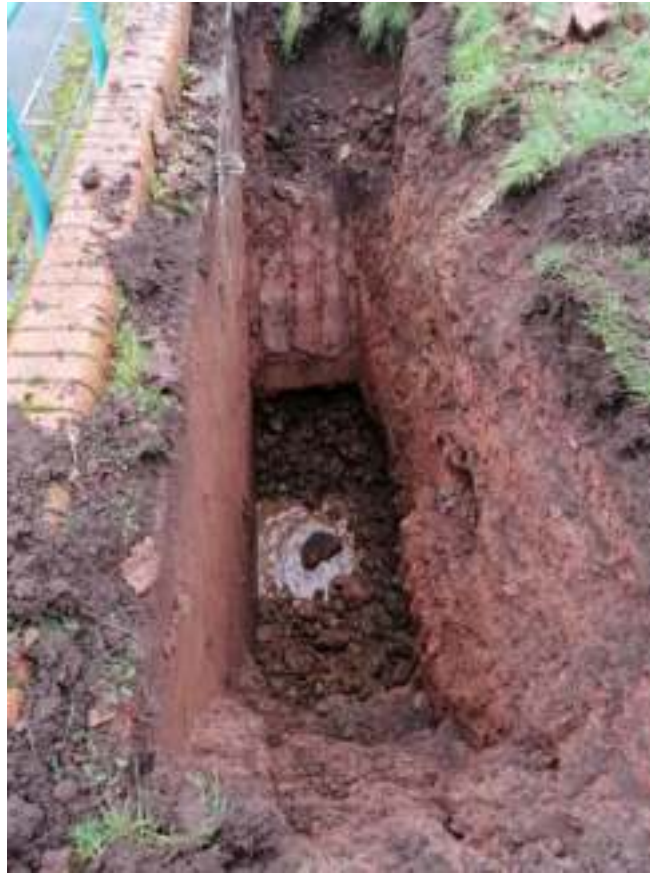
TP05 – Retaining wall inspection from SE side.
