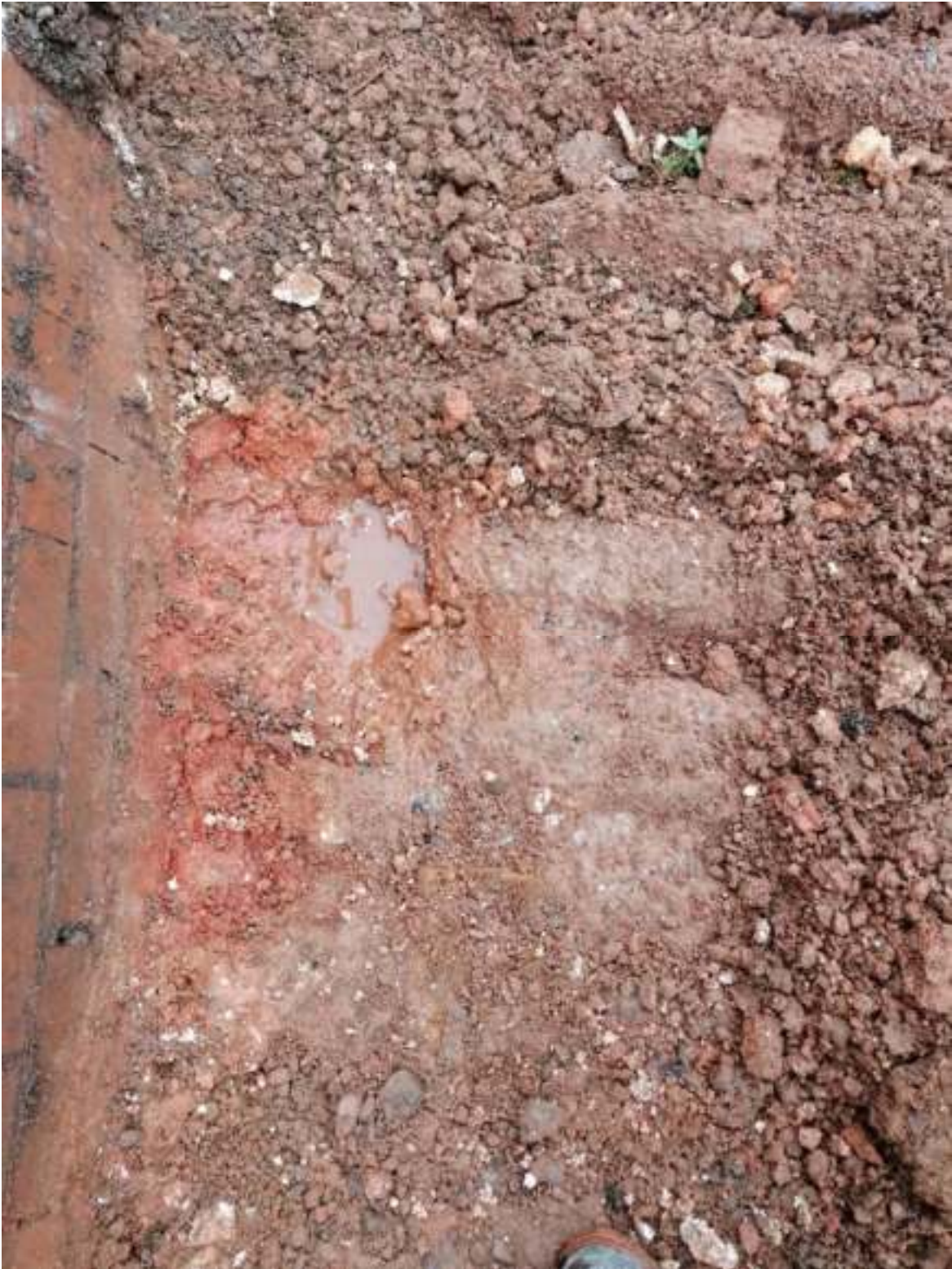
TP04 – Retaining wall footings from the NW side.
