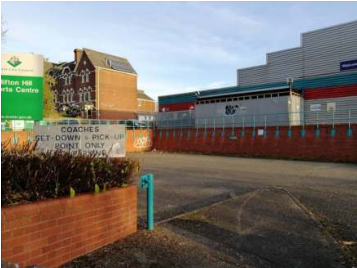
Bottom Car park – Looking SW.
