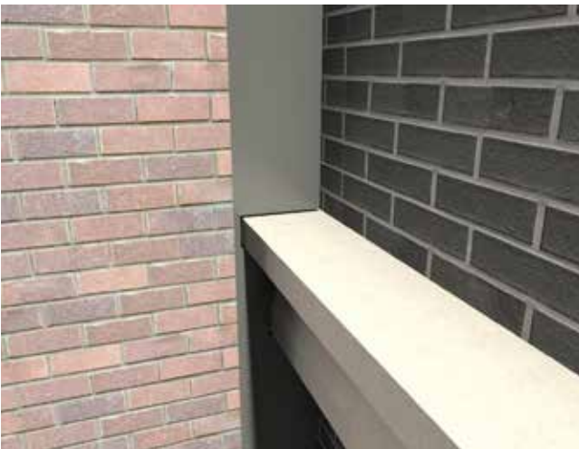
The buildings will connect with a light touch. A recessed metal flashing panel will prevent detritus from collecting between the two buildings.
