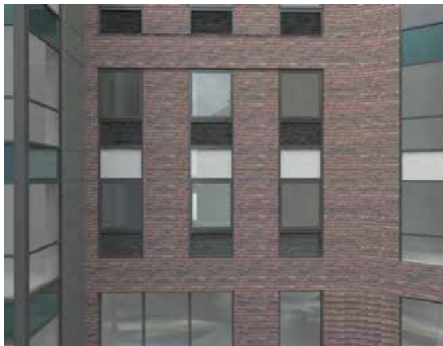
Connecting the windows with spandrel panels and recessed brickwork helps to distort the scale of the building, linking it with both the smaller, more residential, scale of Longbrook Street and the larger, commercial scale of the city centre.
