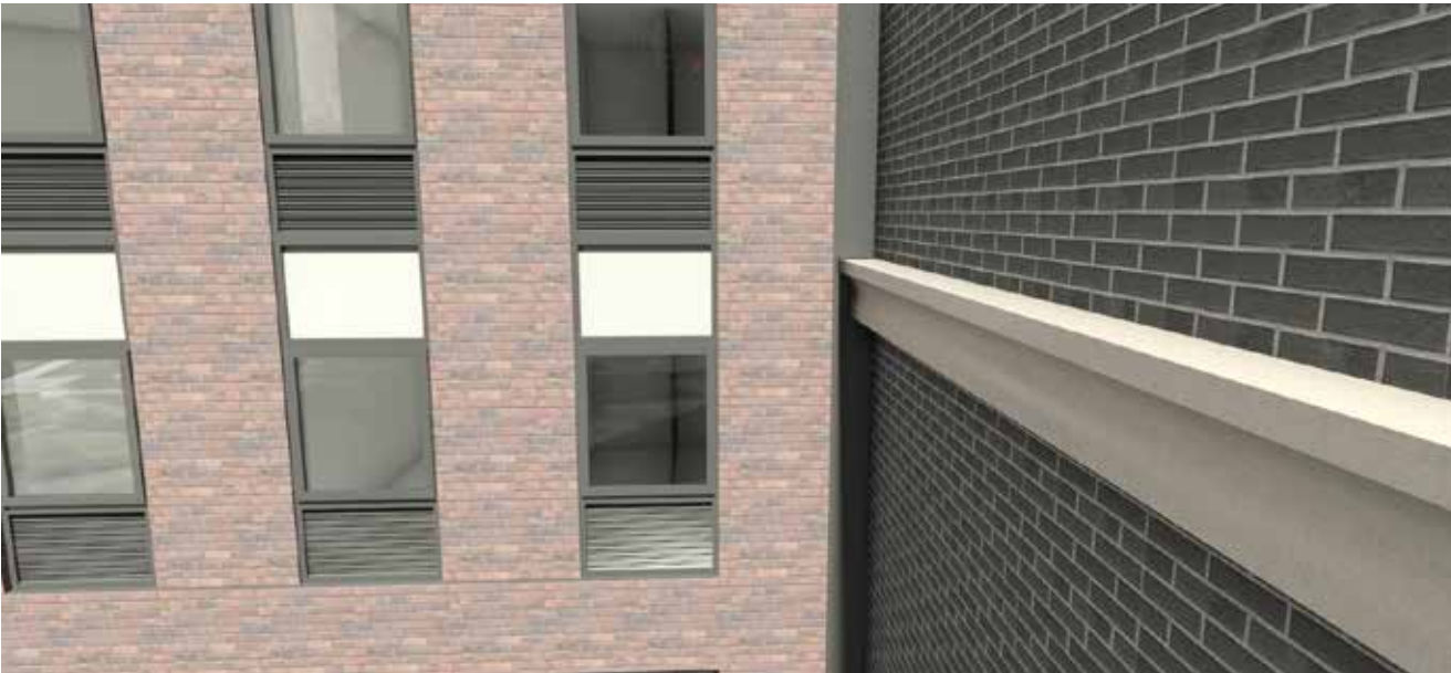
Continuing the white limestone frieze on the John Lewis building in white spandrel panels is a subtle but effective design detail helping to provide a coherent and considered street scene.
