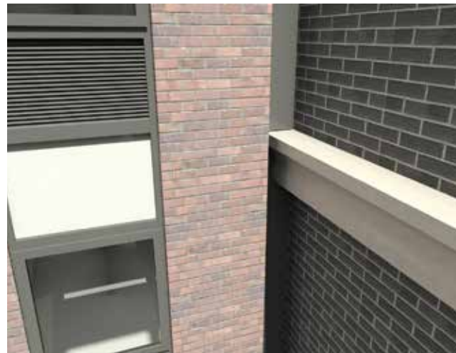
The buildings will connect with a light touch. A recessed metal flashing panel will prevent detritus from collecting between the two buildings.
