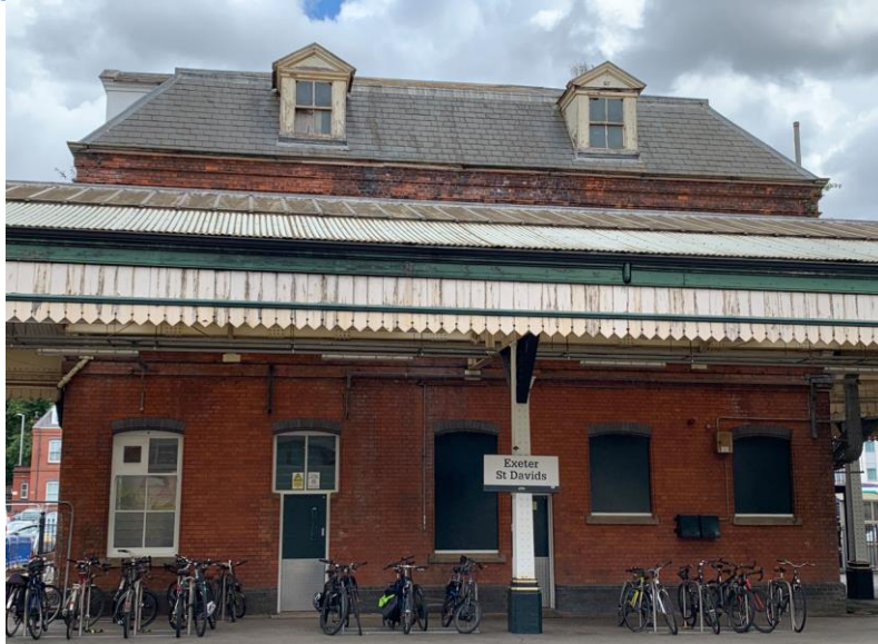
Figure 2 and 3: Building to be demolished
