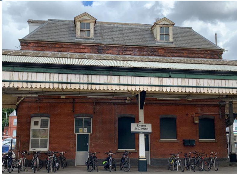
Figure 2 and 3: Building to be demolished
